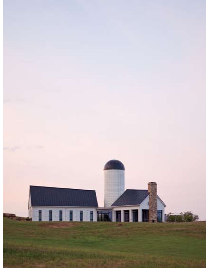
LOCATION. LOCATION Above: The RdV compound, complete with sleek faux grain silo, vat room, and wine cellar. Opposite: The granite RdV wine cellar, carved out of a hillside.
